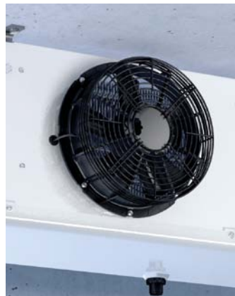
SP 23 = ESM-Motor [EC Technology]
